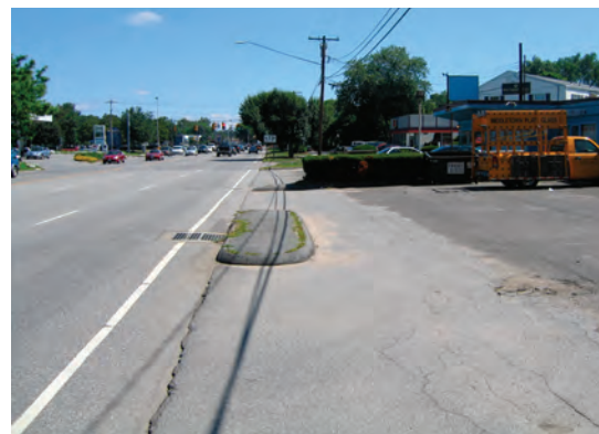
The above example is typical of the many continuous curb cuts along Route 1 in Old Saybrook. As can be seen in the images below, such a landscape is inhospitable to pedestrian traffic.
