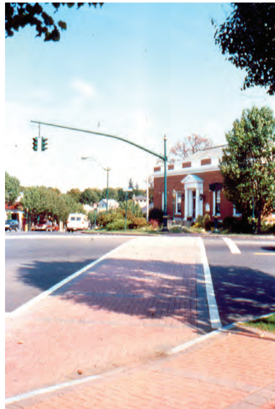
Clearly marked cross walks incorporating a change in surface material such as above and to the right not only make cross walks easier to locate, but also serve to slow down vehicles, making the crossing safer for pedestrians and calming traffic in general.
